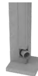
Wasseraustritt Pfostenecke
